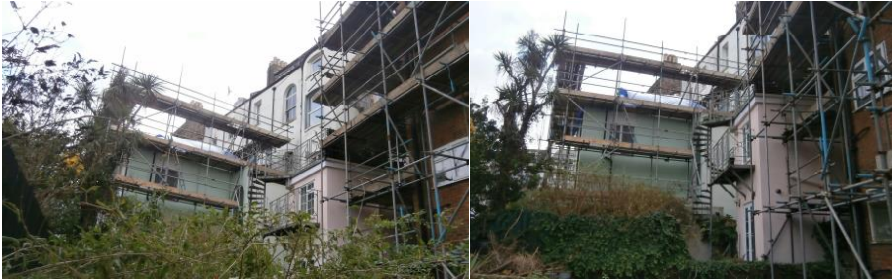
Looking East at Side Elevation of Rear Addition
